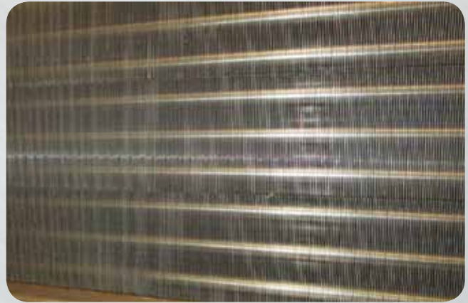
Picture of a coil from a food processing facility, removed to be repaired after nine years in production
